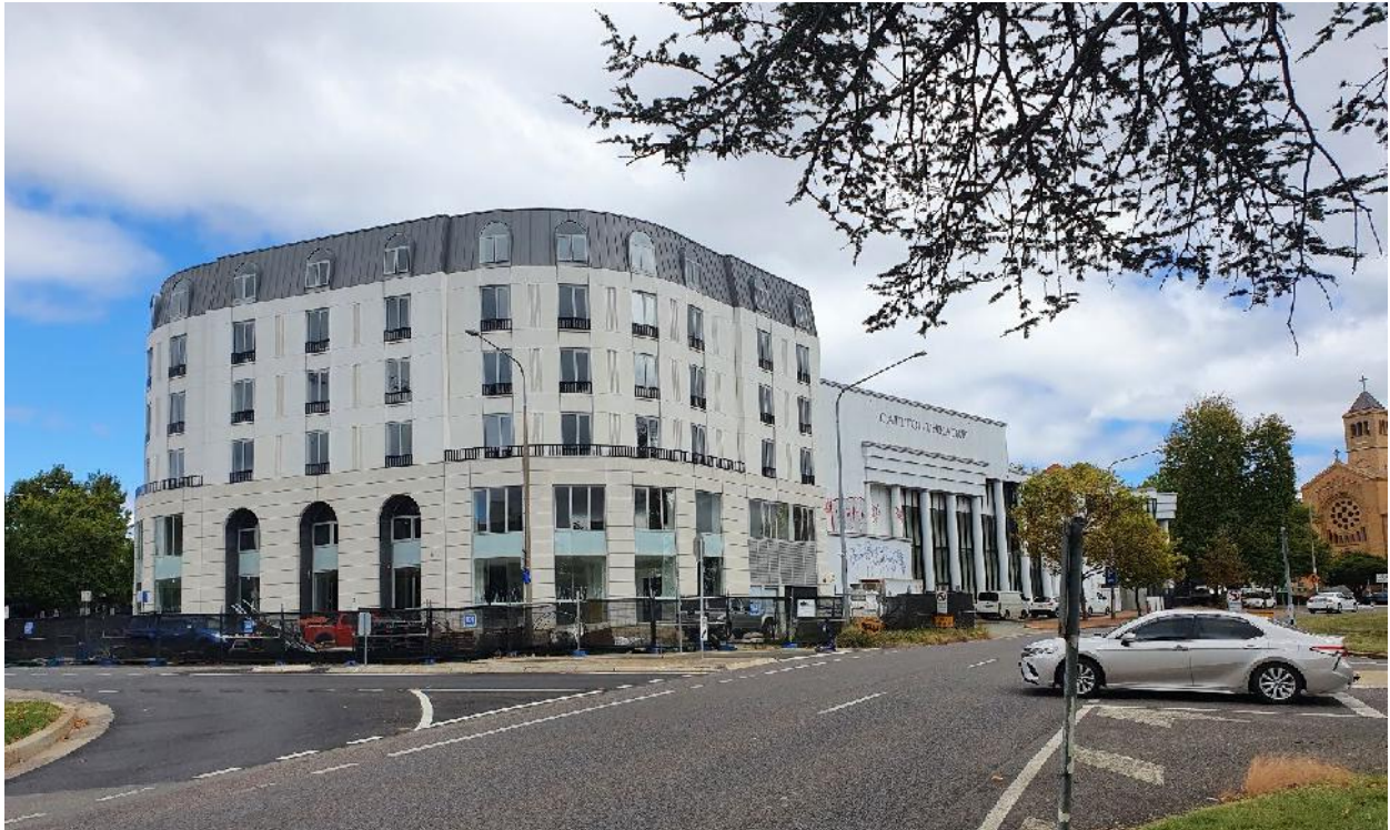
Stage 1 of Capitol Hotel on 6 April 2022, before the start of Stage 2.
